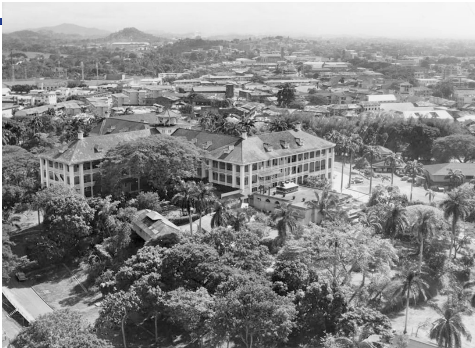
13-K-3 (15) A Tivoli Guest House, Ancon, Canal Zone. June 1, 1956.
