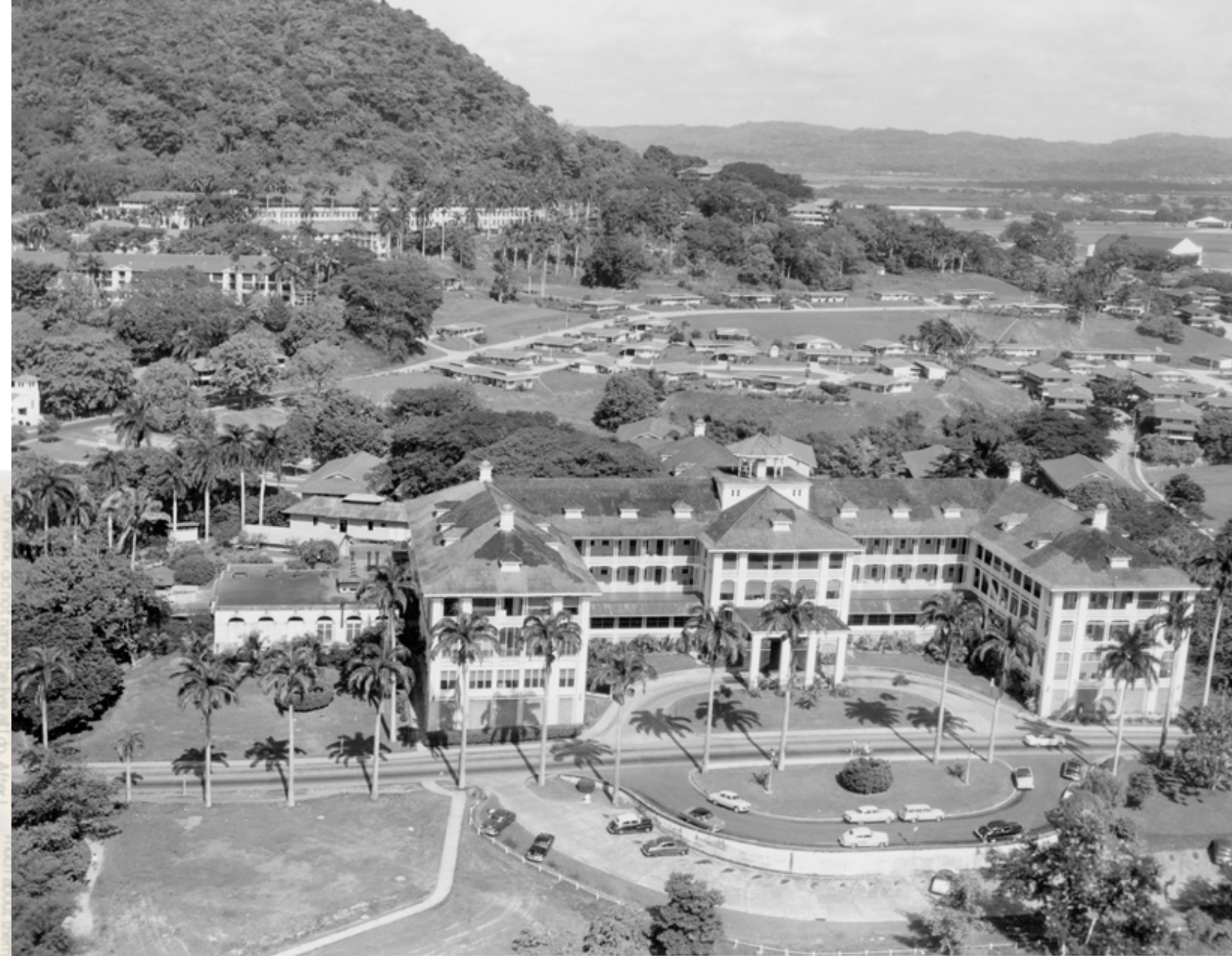
13-K-3 (15) C Tivoli Guest House, Ancon, Canal Zone. June 1, 1956.
