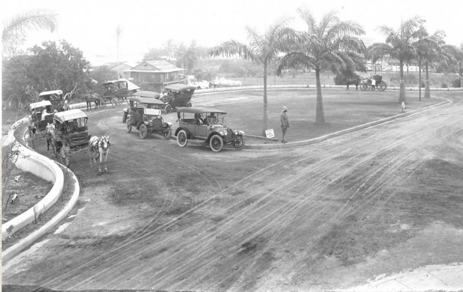
273-J. Tivoli Hotel, Ancon, C.Z. View from north wing, looking southwest. Jan. 16, 1914.
