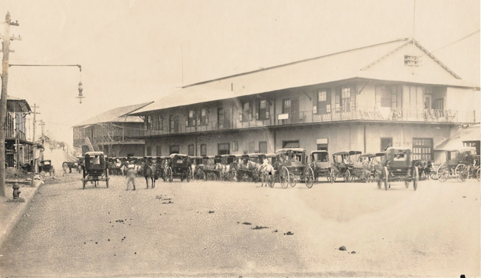
169-A. - Central Ave. Pavement completed. P.R.R. Depot, Panama.
