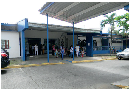
Hospital de Chepo
