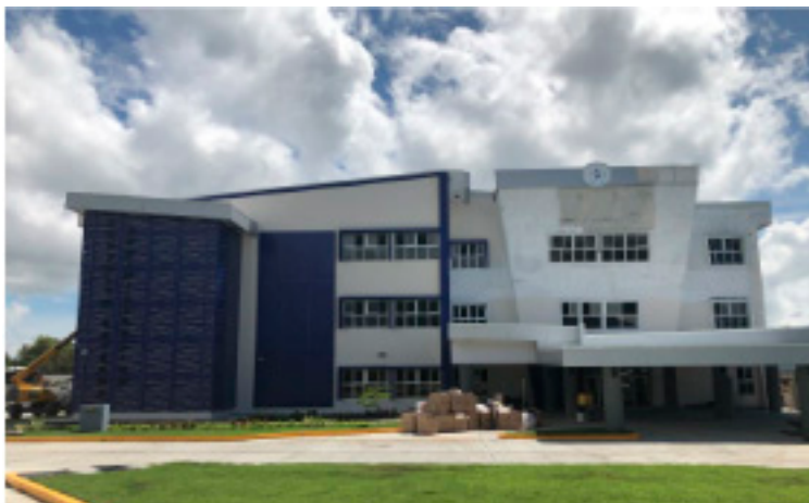
Hospital de Puerto Armuelles
