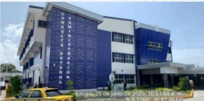
Hospital de Puerto Armuelles
